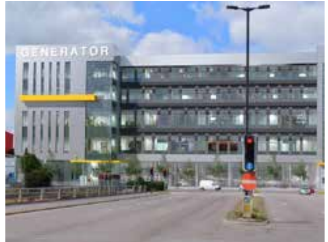
The Generator - front view
