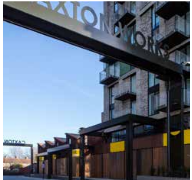
Caxton Works_ External View
