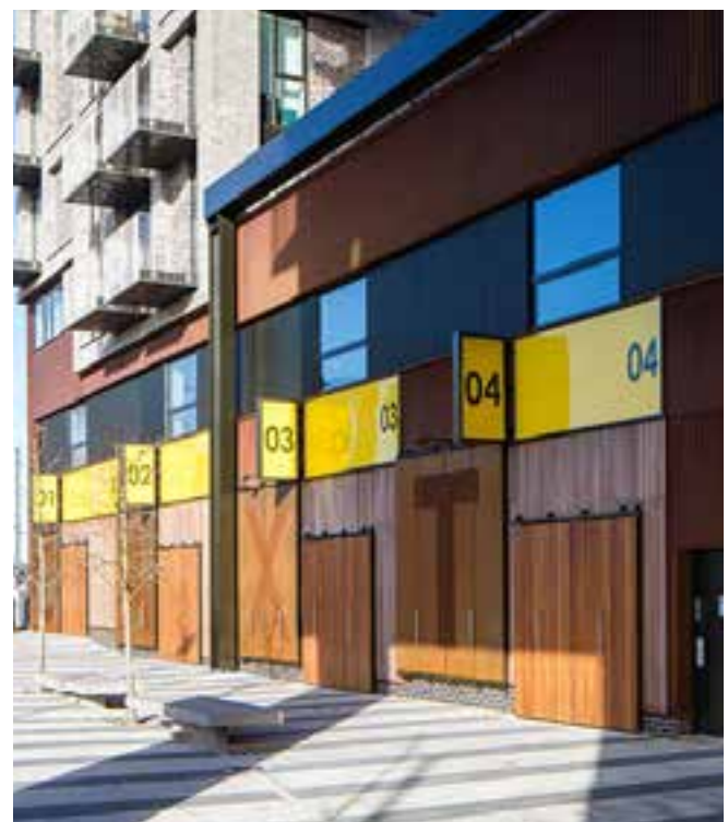
Caxton Works_ External View
