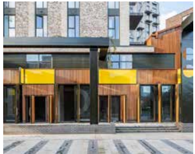
Caxton Works - Central Yard View
