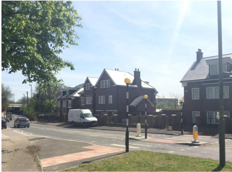
Figure 13: Churchill Place properties fronting Bunns Lane
