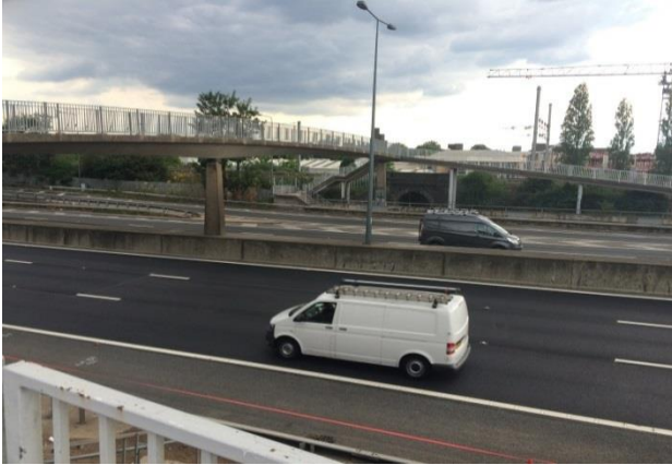
Figure 9: Pedestrian bridge over M1
