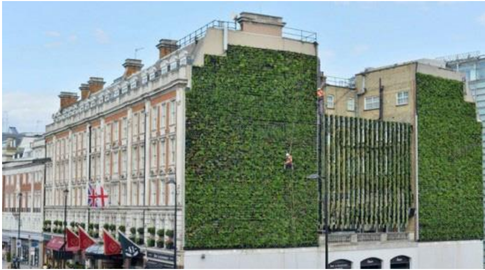
Figure 42 Example of a green wall in Westminster which can act as mental marker for wayfinding
