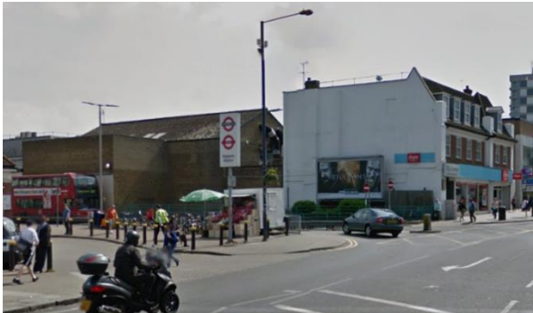
Figure 19 Inactive but visible flank walls
