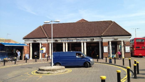
Figure 20 Forecourt to the Station
