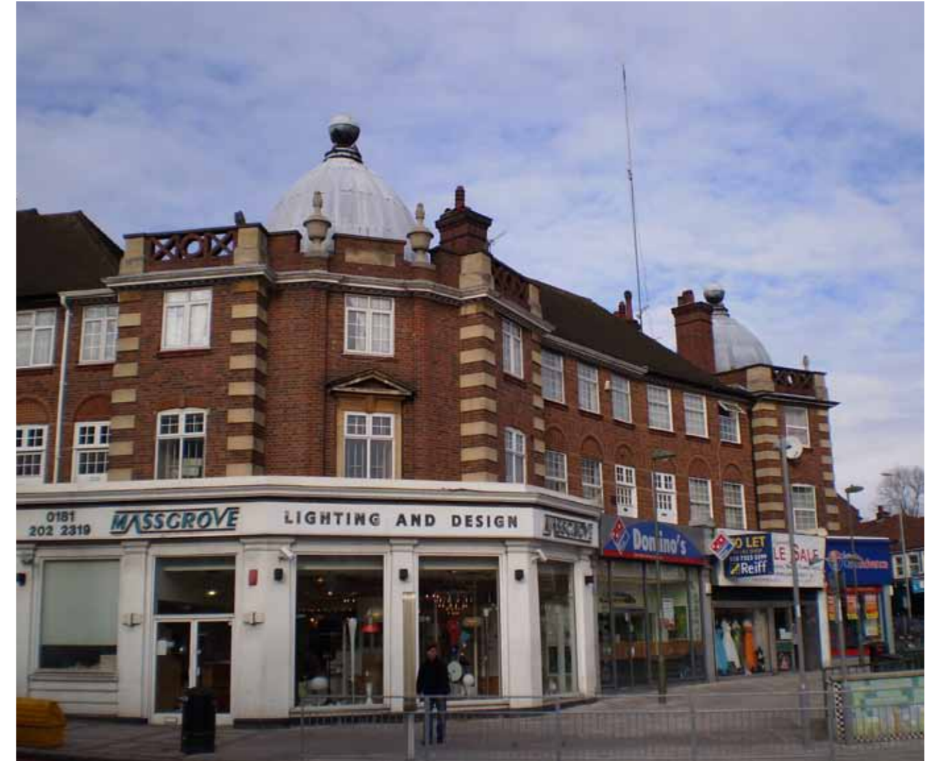
Central Circus in Hendon is an example of a mixed use centre built during the interwar period
