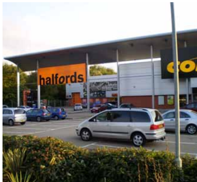
Box development occupies a range of land uses, including retail uses, and is typically surrounded in car parking
