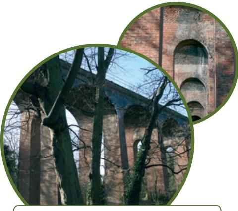
Mill Hill Viaduct's striking high arched brick structure soars high above the Dollis Brook. It was built in the early 1860s for the Great Northern Railway branch to Edgware and has a total of 13 arches. It now carries Tube trains on the Northern Line to Mill Hill East station.
