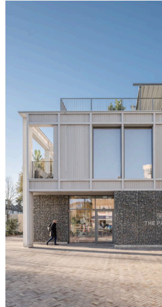
Brent Cross Town Visitor Pavilion, Moxon Architects © Simon Kennedy
