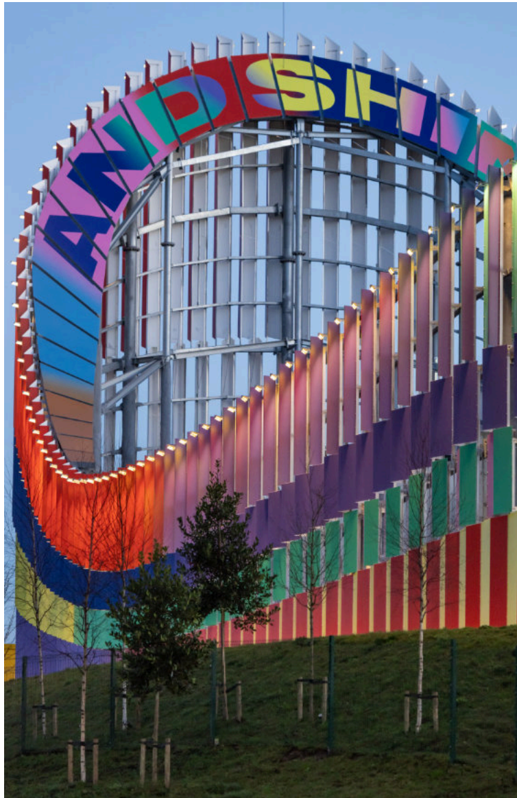
Brent Cross Substation, IF_DO © Jason Hawke
