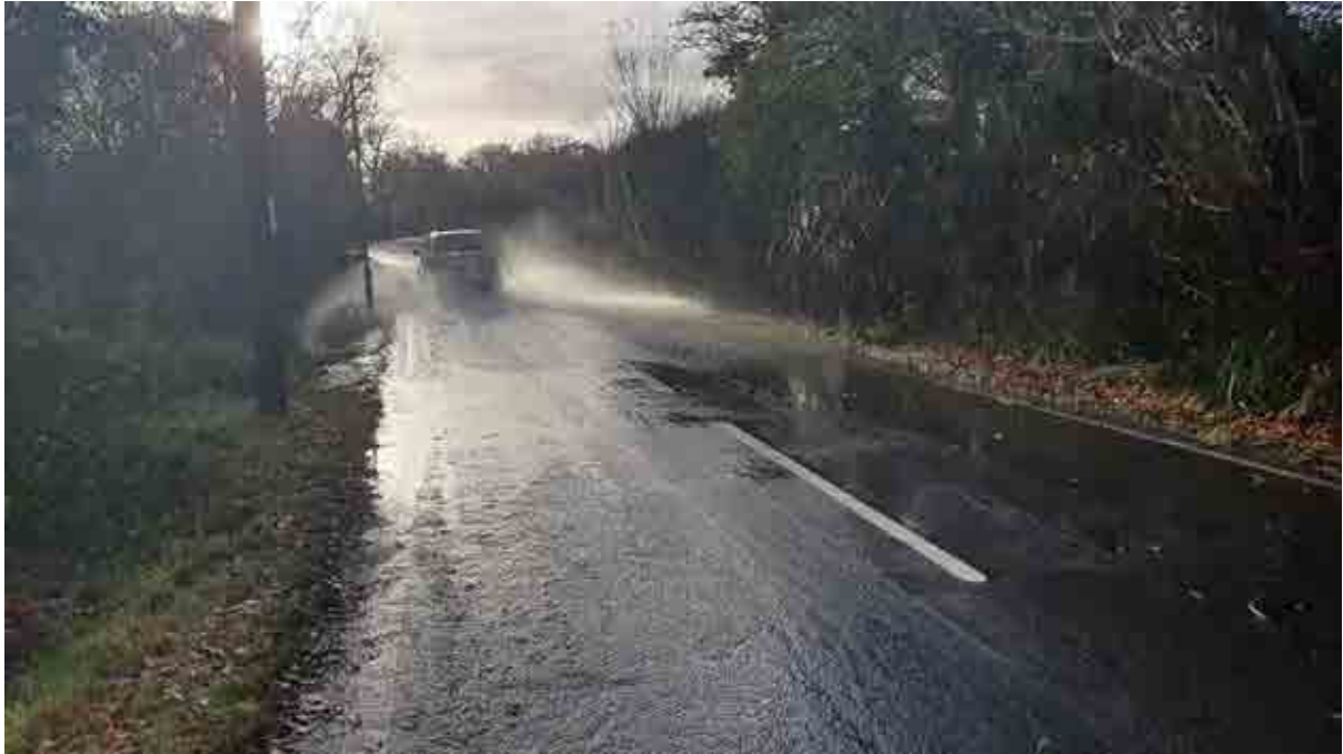
Mays Lane Flooding by Dollis Brook
