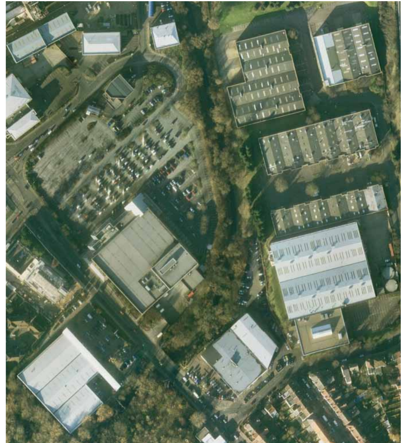
Located in Colindale, the Hyde Estate is a typical example of box development
