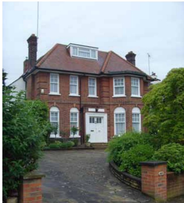
Houses are typically between two and three storeys
