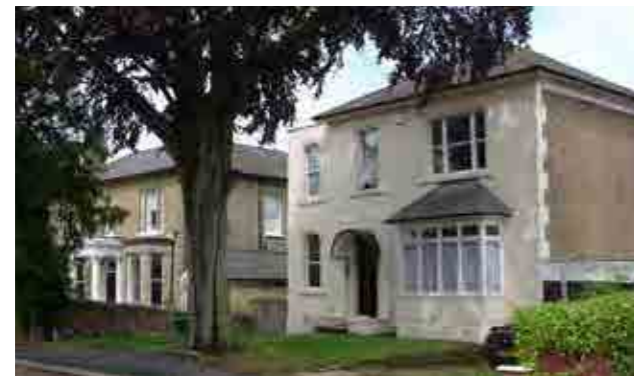
Period buildings have been converted to flats
