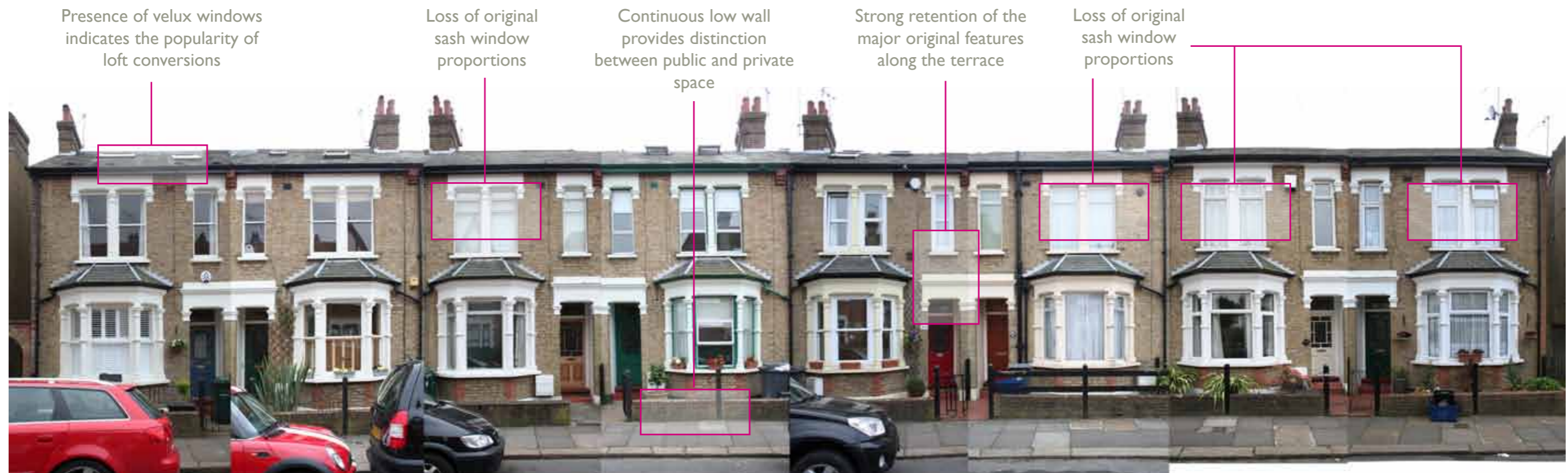
Photographic elevation of The Avenue
