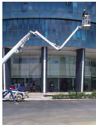
Figure 40: Facade access by MEWP
