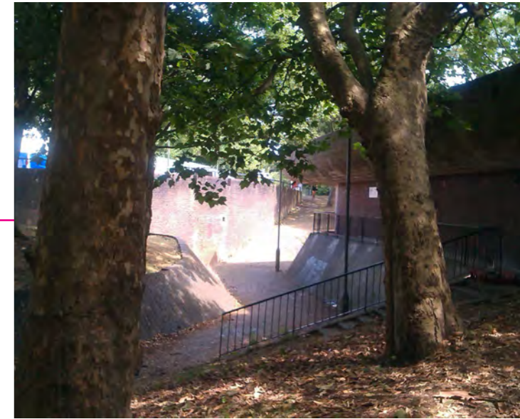
Figure 6: Existing level change surrounding the Energy Centre
