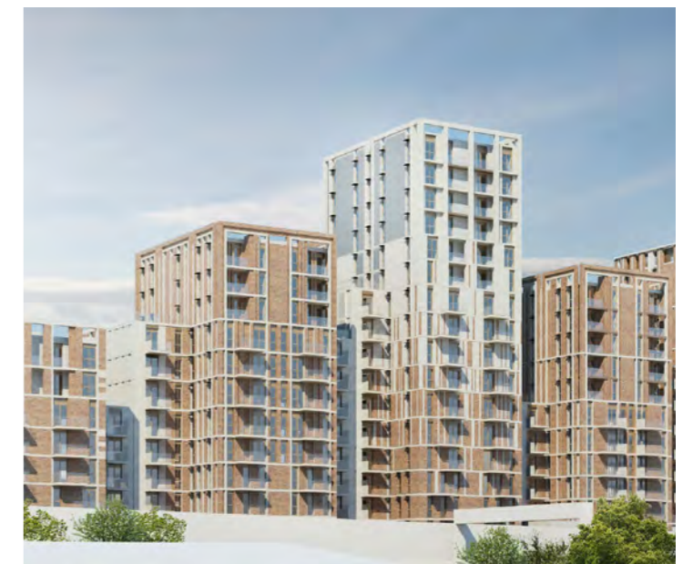
Figure 14: Variable height creates a strong and articulated skyline to the park
