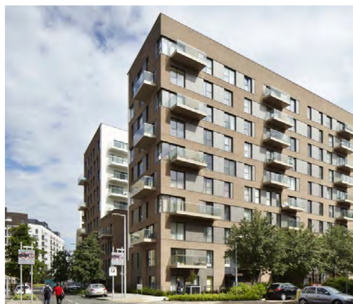
Figure 8: Contrasting lighter toned brickwork to courtyard façades
