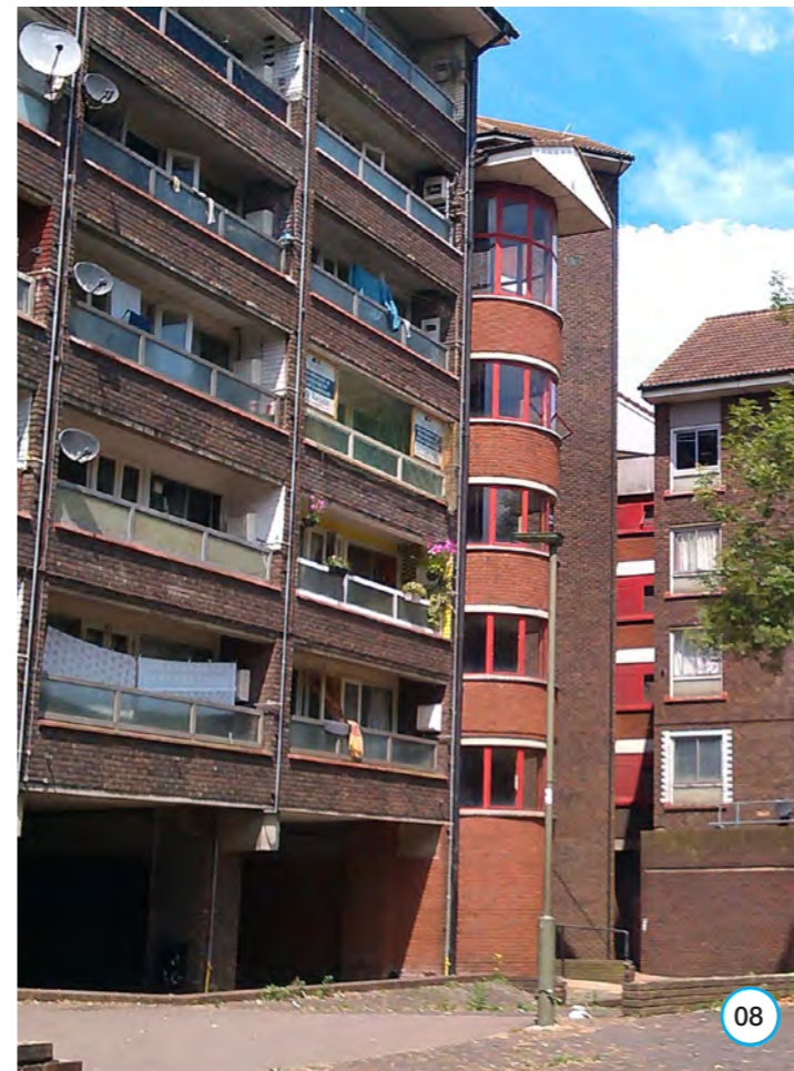
Figure 30: Staircore between 'Nighthawk' & 'Moorhouse'
