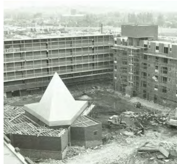
Figure 11: The Community Centre & Concourse under construction (1971)
