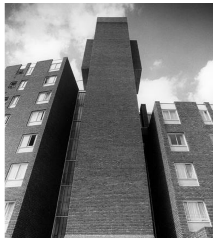
Figure 21: Brick lift core (1975)
