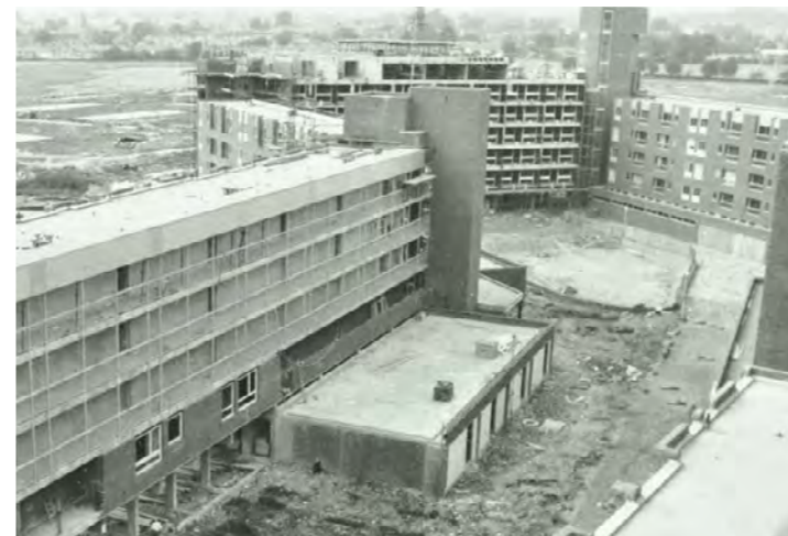
Figure 12: The Concourse under construction (1971)
