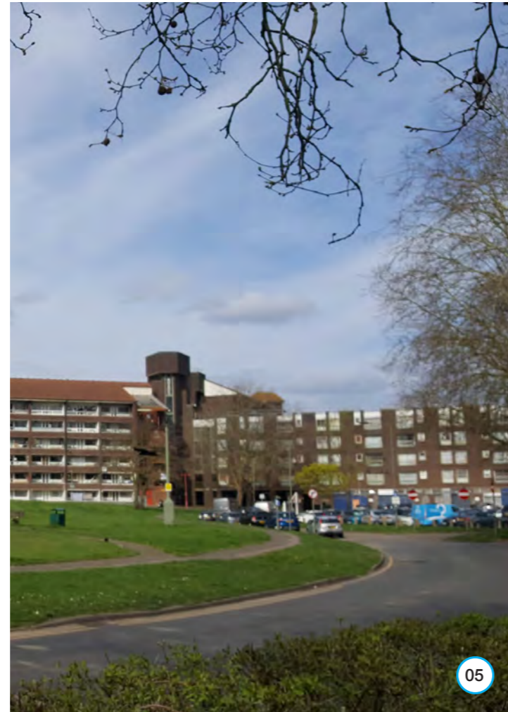
Figure 27: 'Nighthawk' & 'Moorhouse' buildings from Quakers Course
