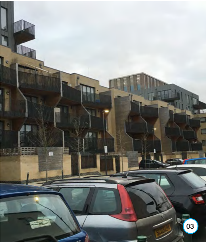
Figure 36: Balconies and parking to the rear of 'Panavia Court'
