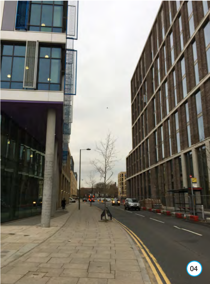
Figure 37: Bristol Avenue between Barnet College & LBB Council building
