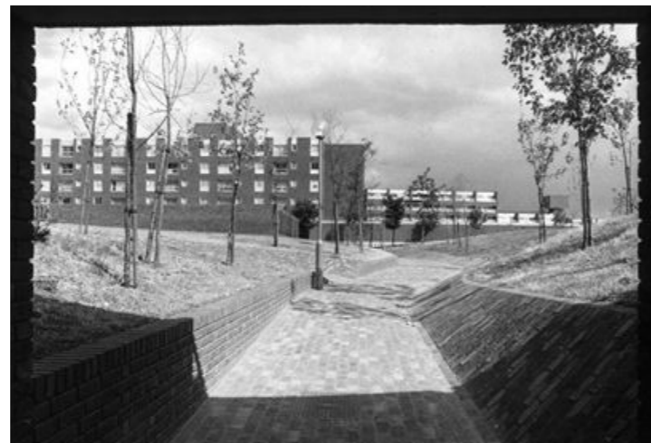
Figure 19: An undercroft pedestrian route (1975)
