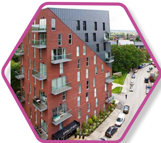
Stonegrove and Spur Road development
