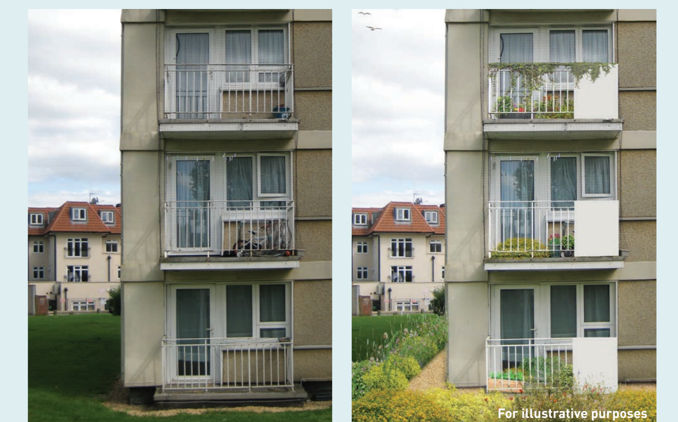
A before and after showing improvements to the balconies
