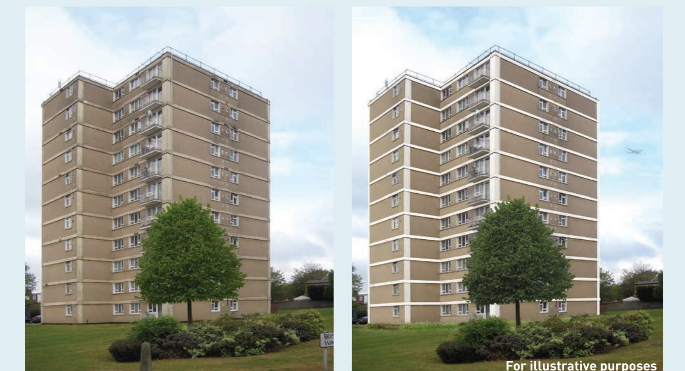
A before and after showing painting of the building's trim
